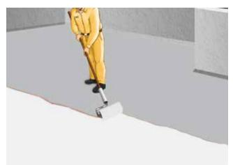
Apply second coat of Dr. Fixit HydroShield PUD Plus without dilution spreading at the rate 0.70/litre/ Sq.mt/ Coat to achieve total dry film thickness of 850 to 1000 microns at forced coverage at the rate of 1.40 /litre/ Sq.mt in 2 coats. Ensure there are no pinholes or air bubbles on the membrane.
