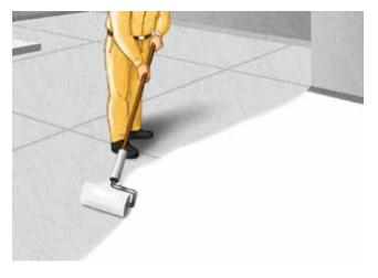
Apply 1<sup>st</sup> coat of Dr. Fixit HydroShield PUD plus without dilution spreading at the rate 0.70/litre/Sq.mt/Coat. Lay a 45 GSM Fiber glass mesh as a reinforcing material which is incorporated in the coating when the first coat is still in wet condition.
