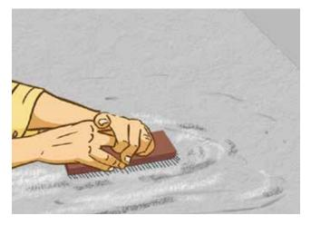
Remove all oil, grease, dust, loose particles and other foreign material. Surface must then be thoroughly washed off with clean water. Substrate MUST be in SSD condition for application of primer.
